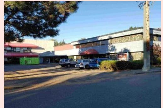
The new Victoria Social Innovation Centre - under renovations in 2017
